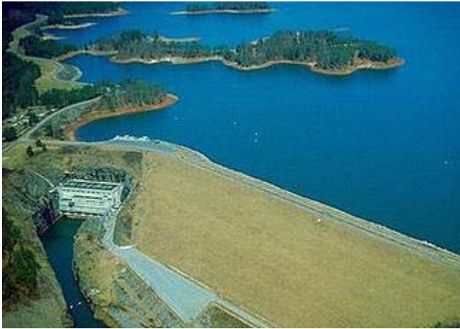
The Buford Dam impounds Lake Lanier in northern Georgia. (Photo courtesy U.S. Army Corps of Engineers )
